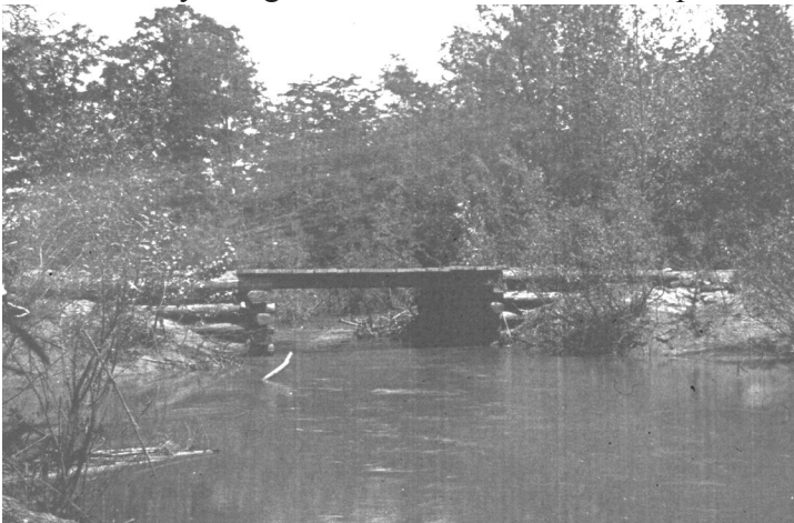
Timber beams on timber abutments. (Unidentified date and location in Posey county.)
