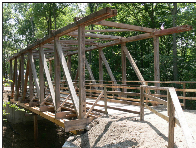
The Pioneer Engineers Club is in process of restoring and relocating Homer's multiple king-post trusses to Caldwell Pioneer Acres in Rush County.
